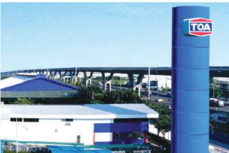
TOA Paint (Thailand) - Samut Prakan
