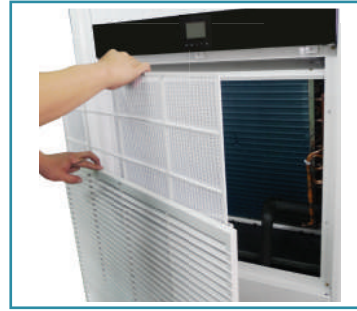
Return air grille and air filter
