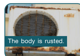
The fins are corroded.
